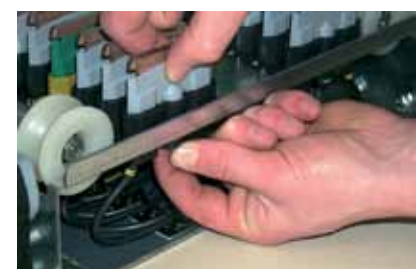
Replacing the carbon brushes.
