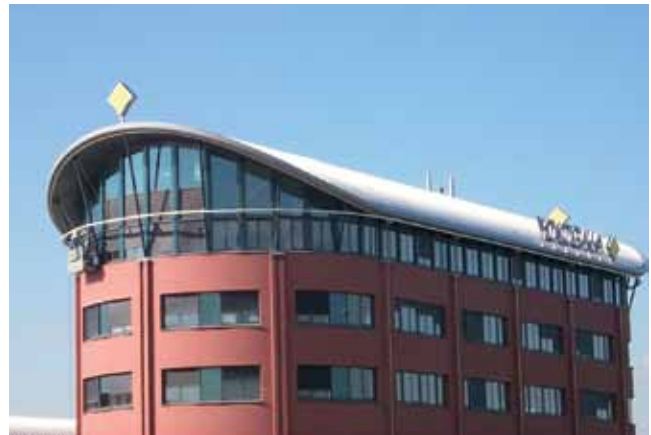
Curved installation for window cleaning equipment
